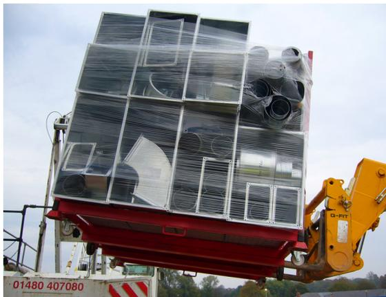
Figure 2 Kit of parts for vent system on mobile stillage
