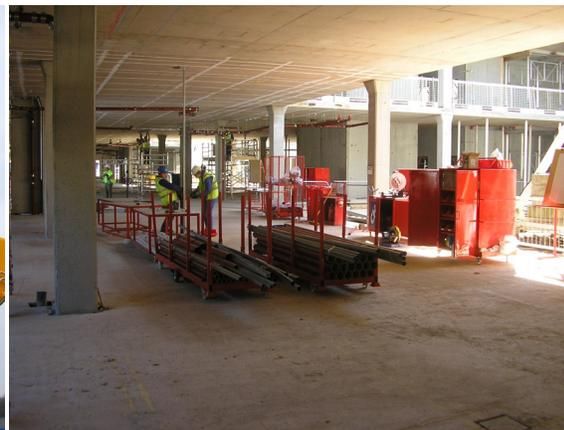
Figure 3 Mobile work cell - drainage crew
