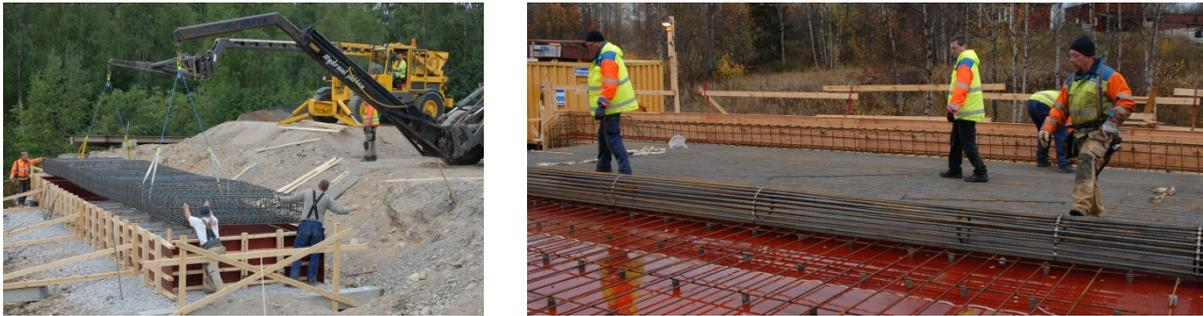
Figure 7: Use of prefabricated reinforcement cages (left) and rebar carpets (right).
